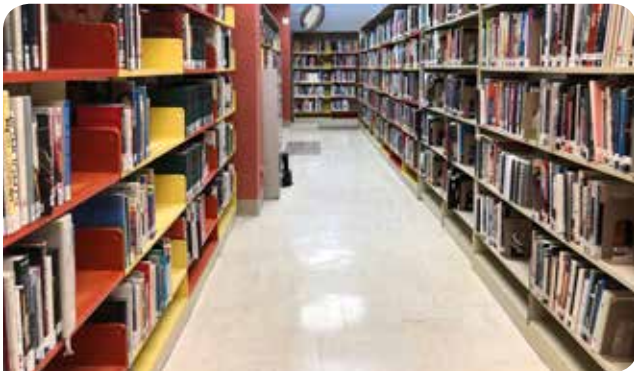
Shelving is not FADS compliant
