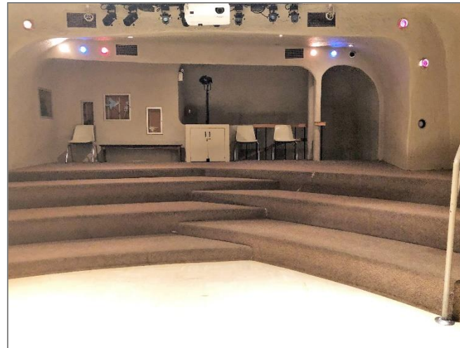
Story room is original to the building, lacks accessibility and the design of the stairs are a tripping hazard
