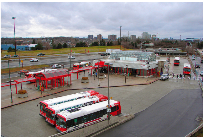
Figure 5. BRT and local bus terminal at St. Laurent Shopping Centre in Ottawa
