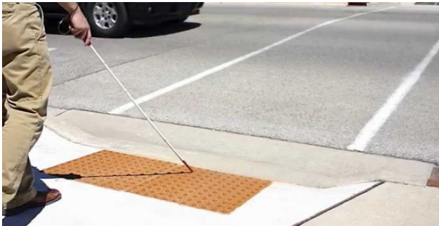
Figure 4. Detectable Warning Strip
