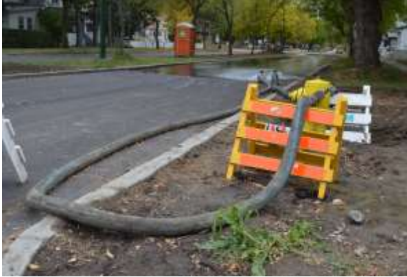
Water system flushing.
