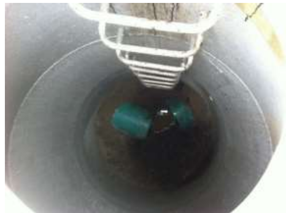
View after installation.
