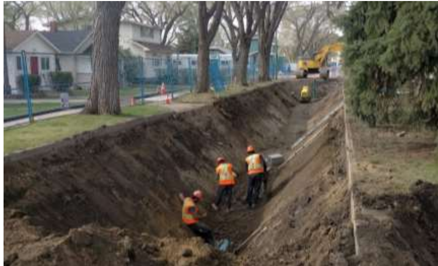
Water main installation.
