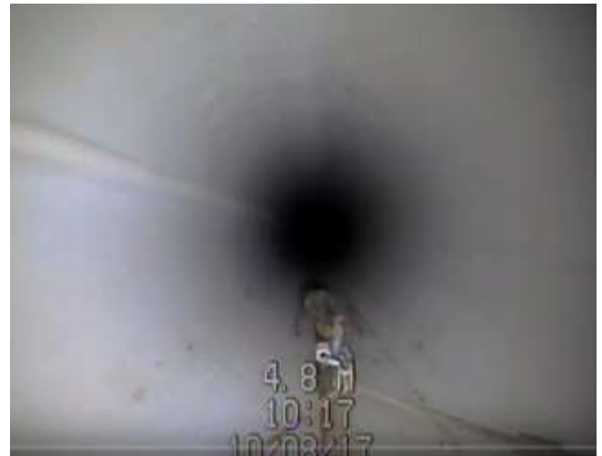
300 mm cast iron water main post-lining.
