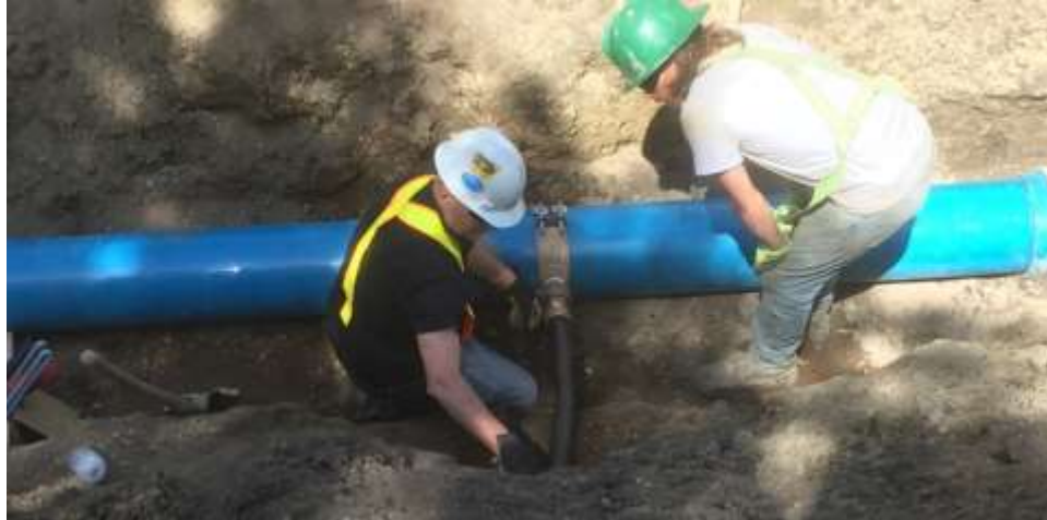
Installation of new water service connection pipe to new water main.
