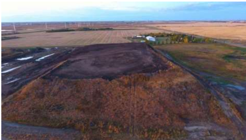
The topsoil stockpile during construction.
