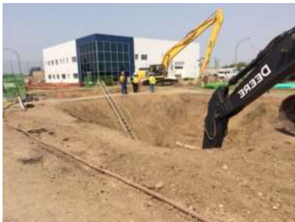
Installation of manhole at Buckle/Fletcher Road Intersection.
