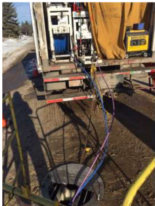
Final CCTV inspection.
