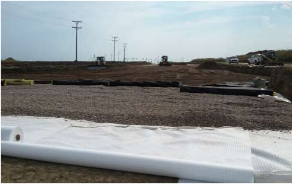
Intersection of Market Drive and Zimmerman Road looking south.
