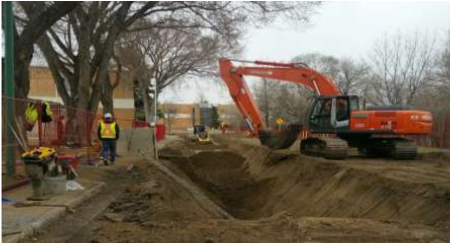
Spadina Crescent West during water main Installation.
