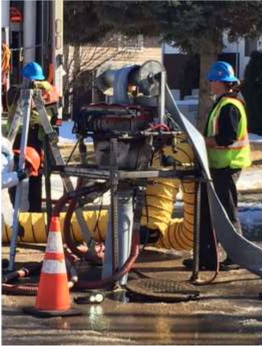
200 mm sewer main CIPP liner insertion.
