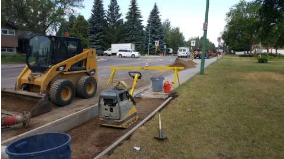
Concrete base preparation.
