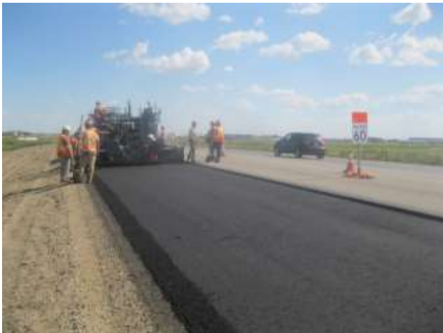
71st Street base gravel compaction.
