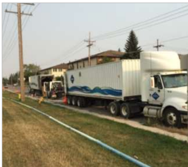
Contractor setup for installing CIPP liner.
