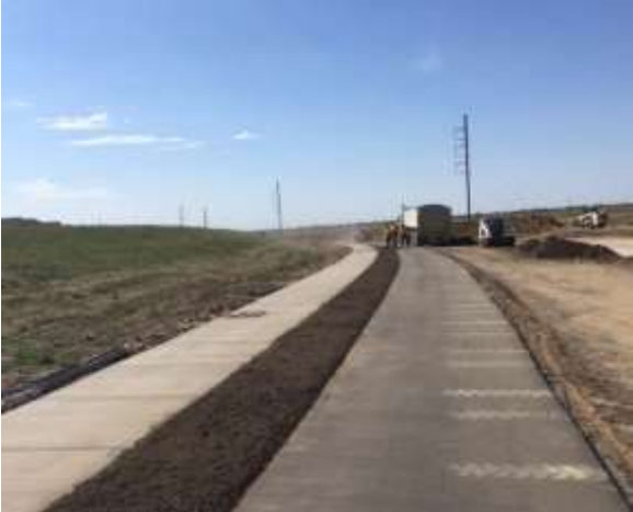
Completed sidewalk and bikeway along the south side of Fedoruk Drive.
