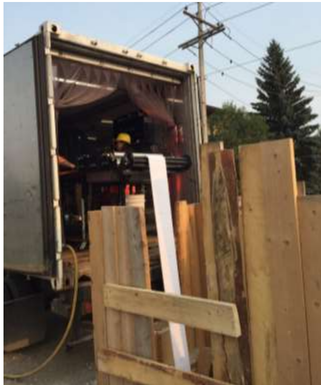
CIPP Liner being pulled into existing water main.
