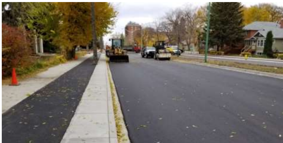
New sidewalk, cycle track, curb, and roadway surface on Victoria Avenue.
