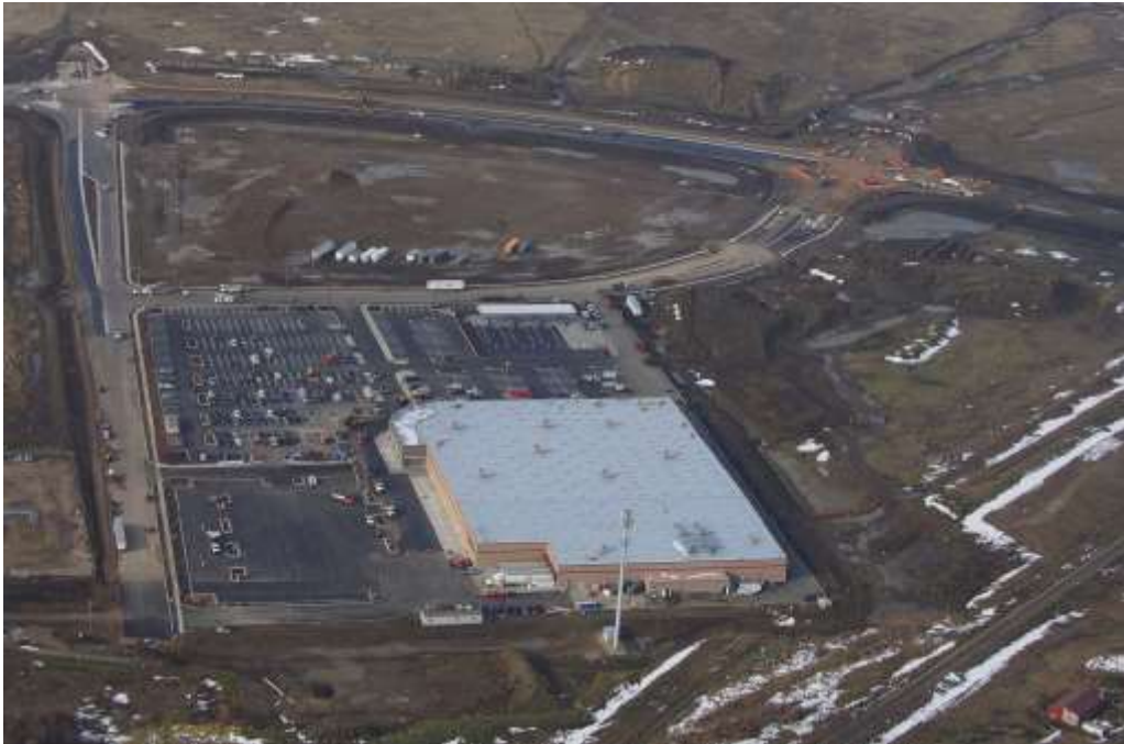
Intersection of Zimmerman Road and Highway 16 looking west.
