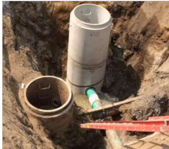
New manhole at Fletcher Road and Buckle Avenue.
