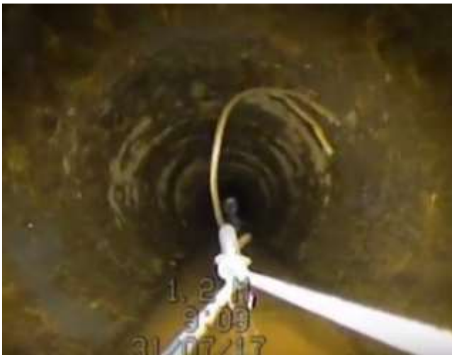
300 mm cast iron water main pre-lining.
