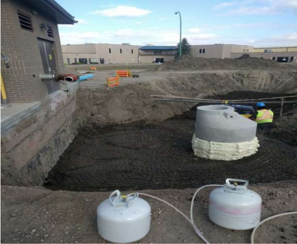
Installation of manhole close to Fletcher Road lift station.
