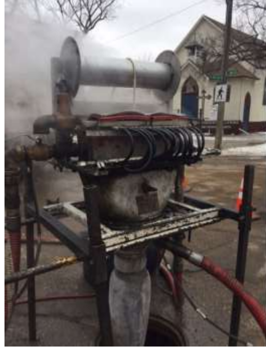
200 mm sewer main CIPP liner insertion.
