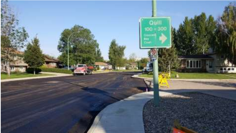
Tack coat following milling.
