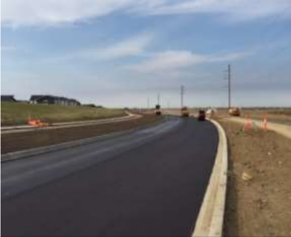
Asphalt paving on Fedoruk Drive.
