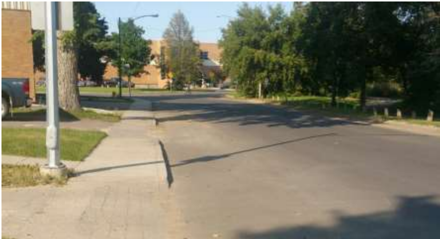
Spadina Crescent west after completion.
