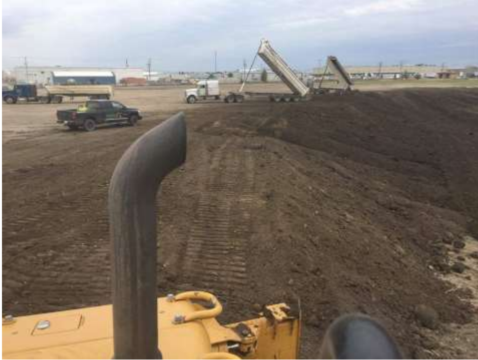
Trucks dumping topsoil into the Hudson Bay borrow pit.
