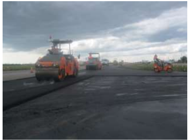
71st Street base gravel compaction.
