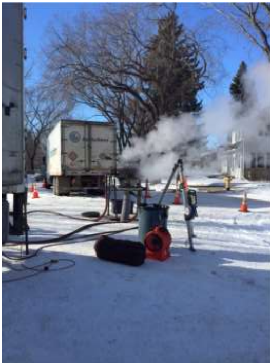
Curing CIPP liner.
