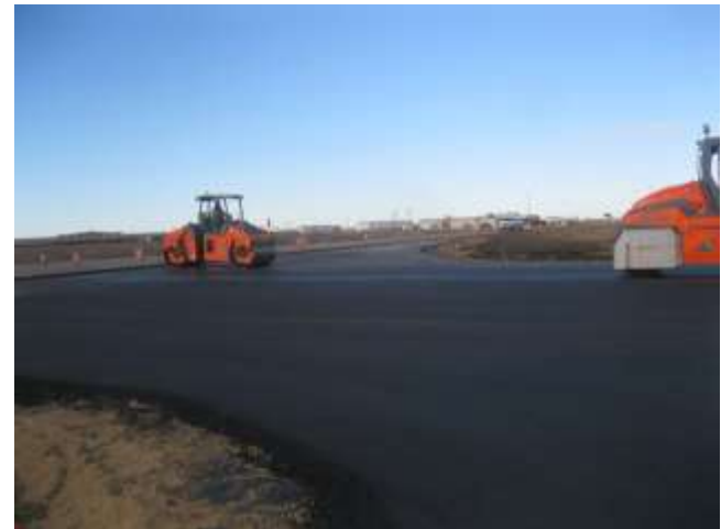
Finished Pavement at 71st Street and Highway 16.
