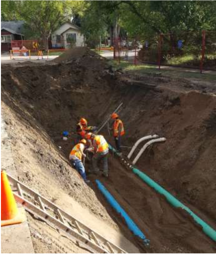
Both water and sewer main replacement.
