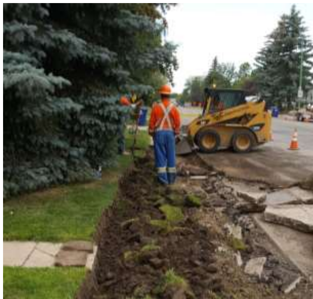
Concrete removal.
