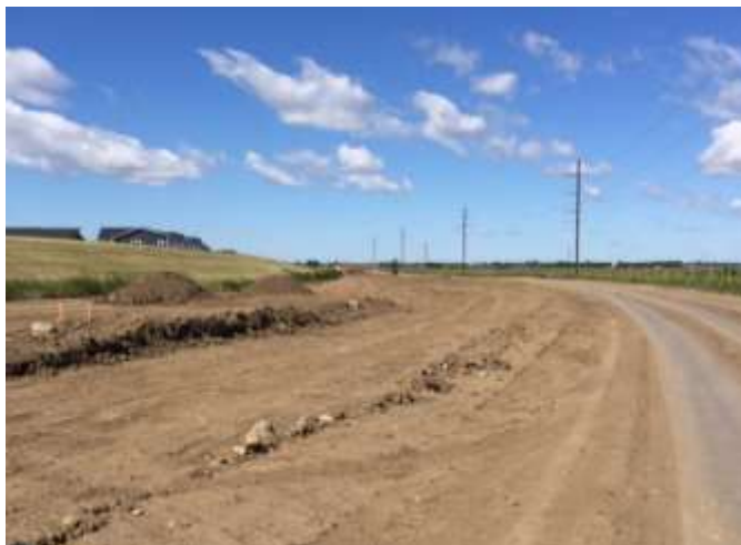
Site conditions at the start of construction.
