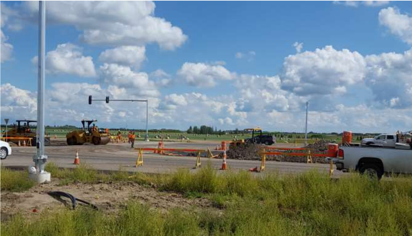
Intersection of Zimmerman Road and Highway 16 looking south.
