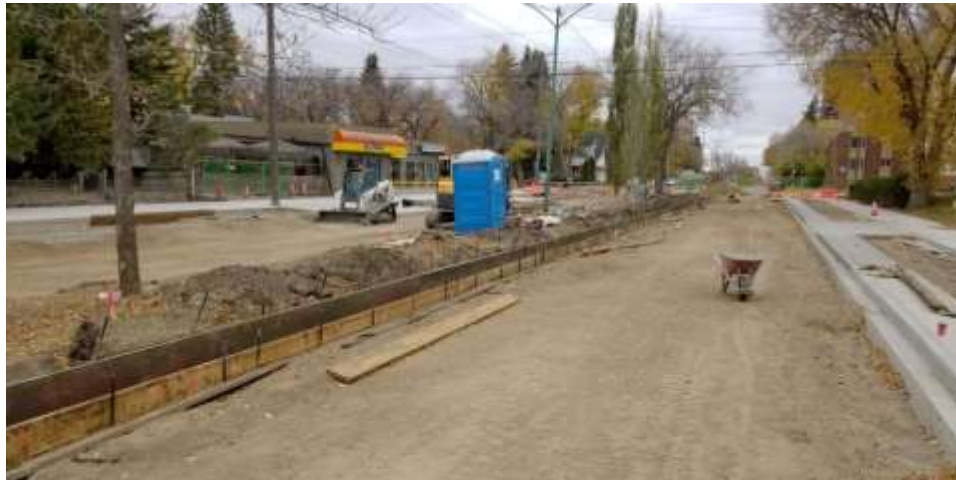
Reconstruction of Victoria Avenue.
