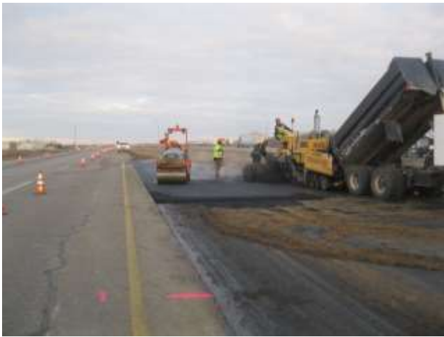
Paving turn lane.
