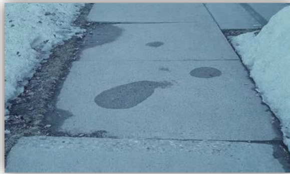
Mud Jacking or Replacement
