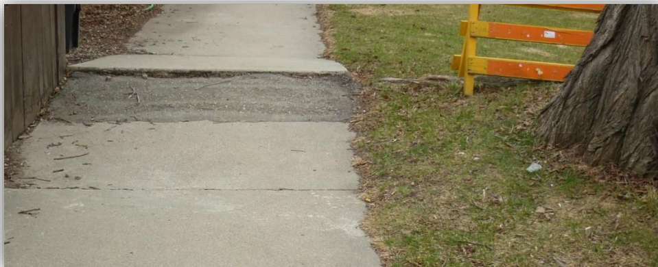
Tree Root – Replacement
