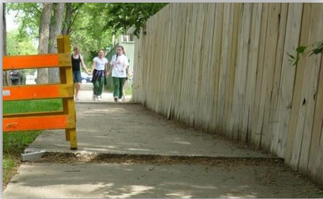
Repair – Grinding or Saw Cut
