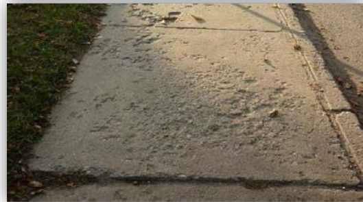
Medium Severity – MG Krete Overlay
