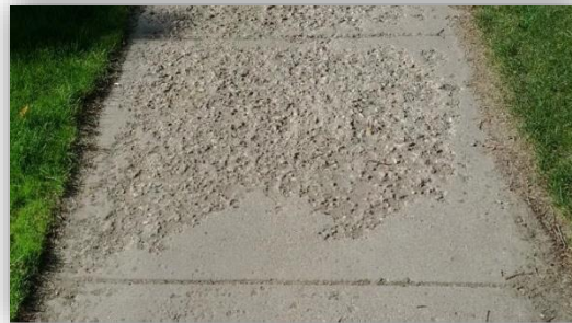
High Severity – MG Krete Overlay
