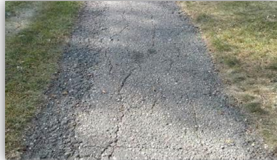
Fair Condition Asphalt Overlay - Replacement
