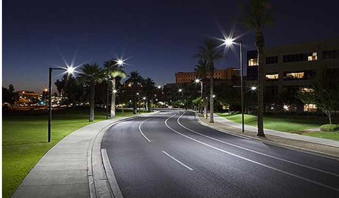
Increasing Roadway Network 2016 = 30 KM added (0.7%)
