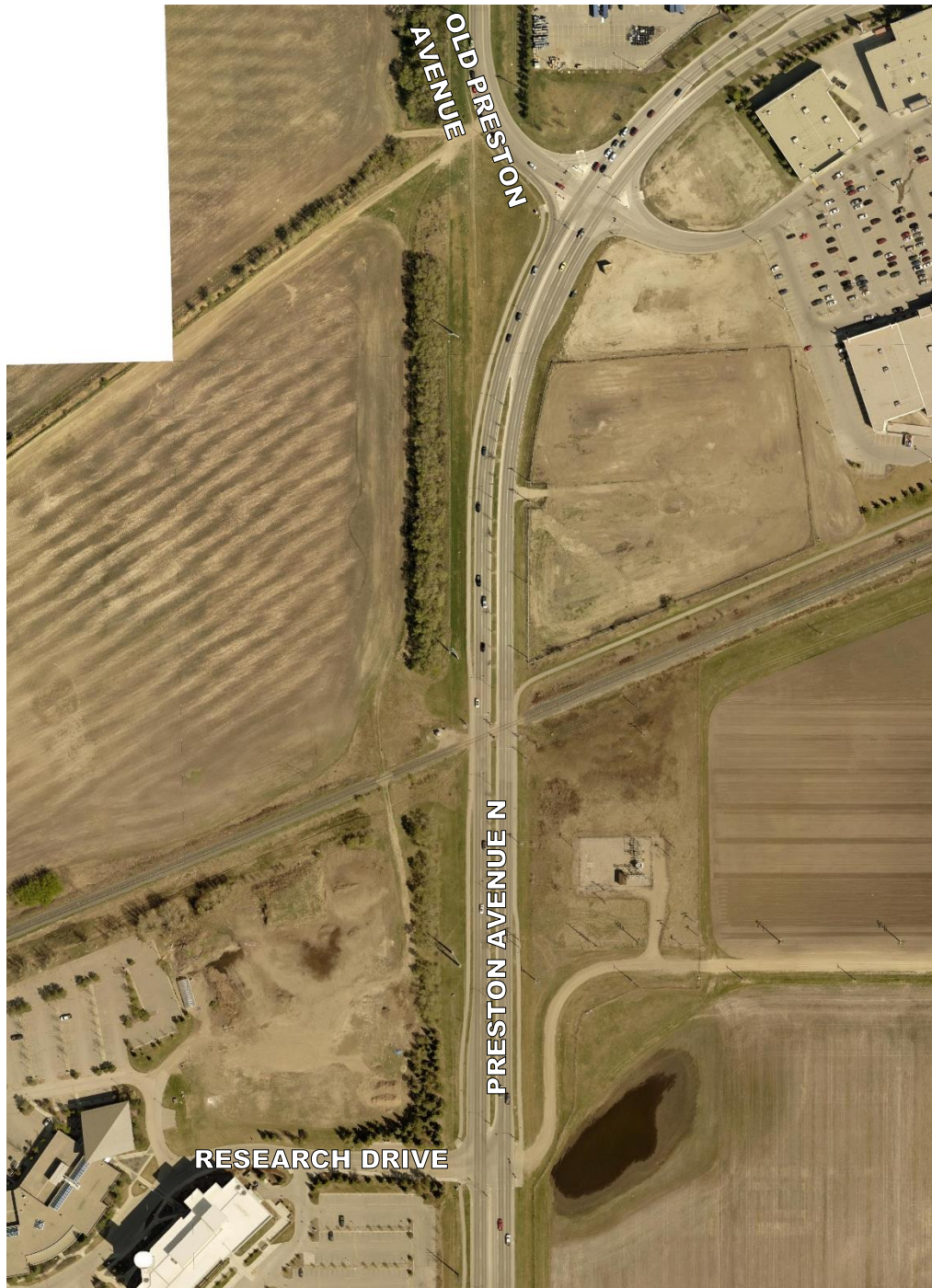
Figure 10: Preston Avenue N @ CP Crossing
