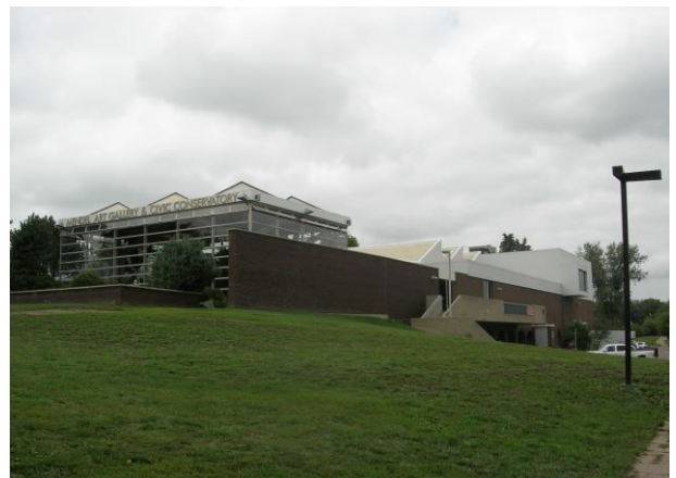
South and East Façades (2015)
