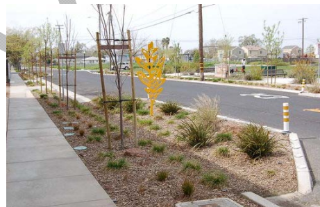
Figure 10: Stormwater bump out example
