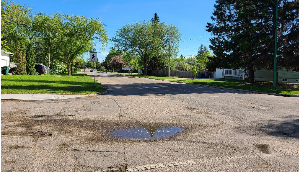
Figure 3.3 Looking South at pedestrian crossing on Victoria Avenue at Isabella Street
