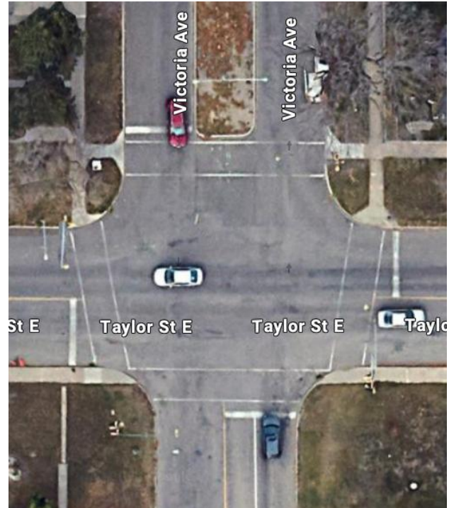
Figure 2.16 Crosswalk Alignment at Victoria Avenue and Taylor Street East
