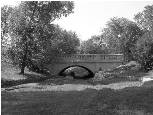
Top: Spadina Crescent Bridge. Source: City of Saskatoon
