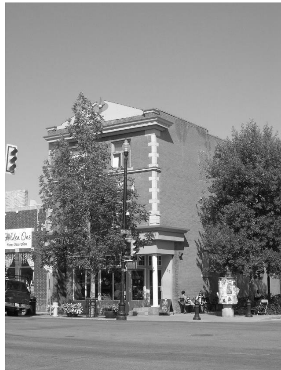
Top: Eaton Block. Source: City of Saskatoon
