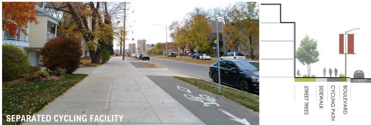
Figure 4: A separated cycling facility, such as on Victoria Avenue in the Nutana neighbourhood.
