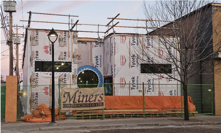
Under Construction – November 2023
