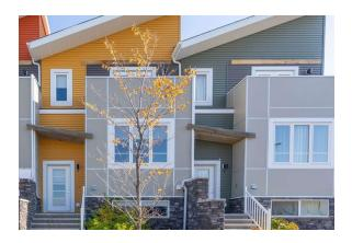
Wall cladding in a single material is not permitted. Durable high-quality materials should be utilized for cladding on all building faces. The use of vinyl products is acceptable on all elevations that are not fronting, any public street or public park, unless it is an approved accent product by Saskatoon Land.
