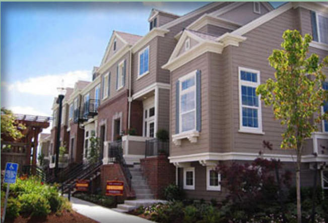
Above: Good examples of buildings interfacing with public street.
