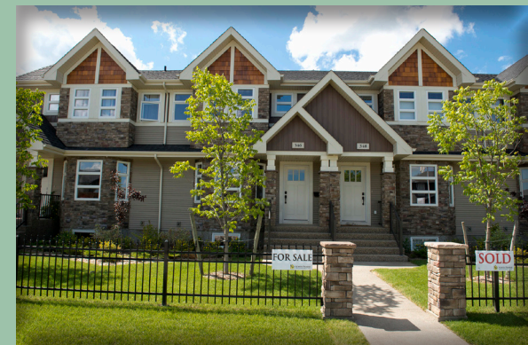
Above: Each of the above images demonstrates a minimum of two exterior cladding materials with sensitively designed proportions.
