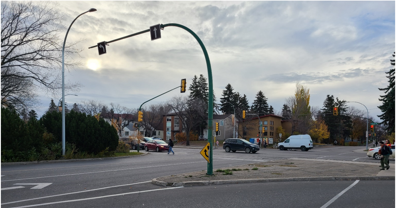
Photo 13 Damaged Double Arrow Sign
