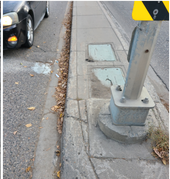
Photo 4 Breakaway Bases
