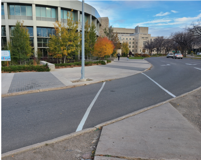
Photo 11 Missing Curb Cuts
