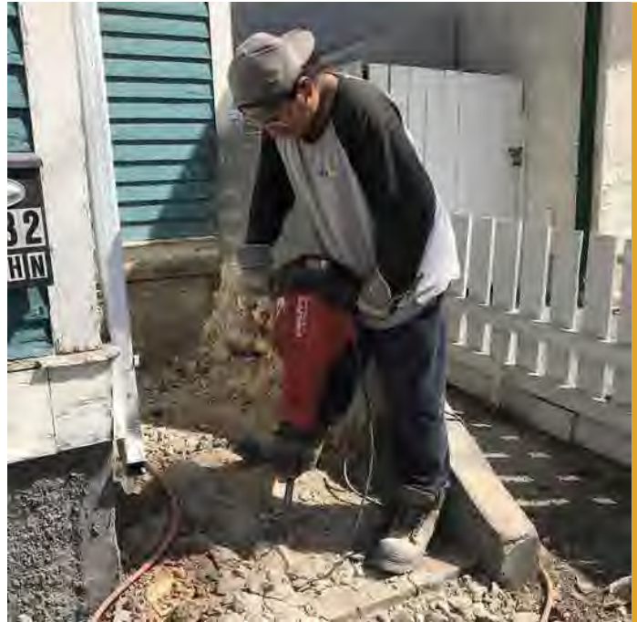
Image 1: Build Up participant demolishing worn concrete steps.
