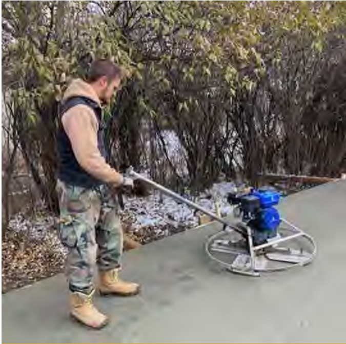
Image 2: Build Up participant training to work with concrete.
