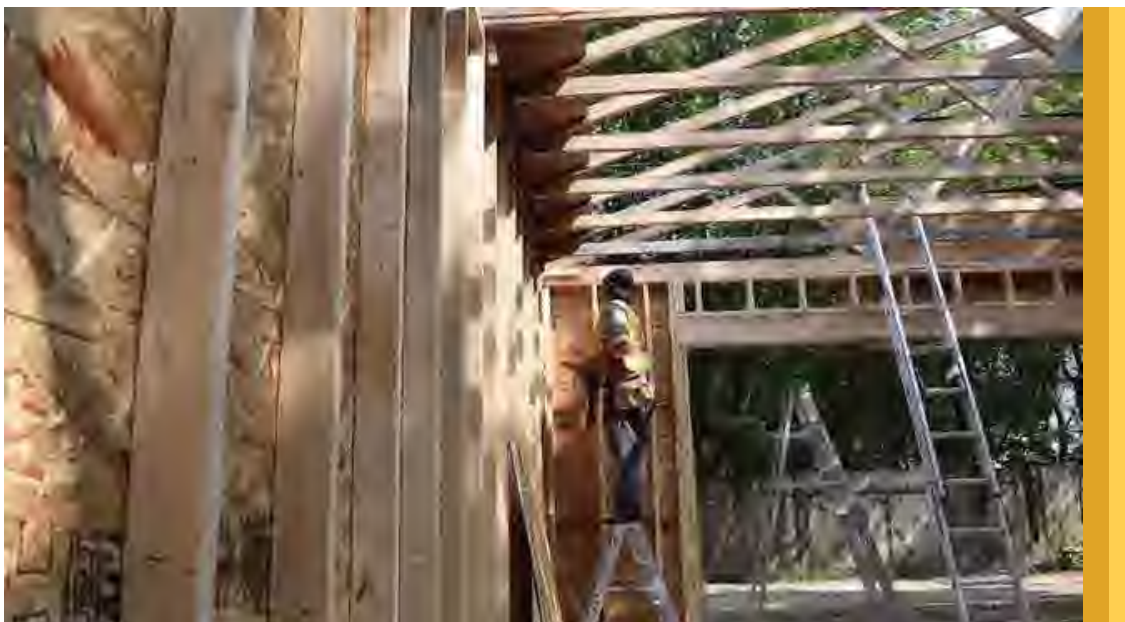
Image 3: Build Up participant putting up rafters in garage.
