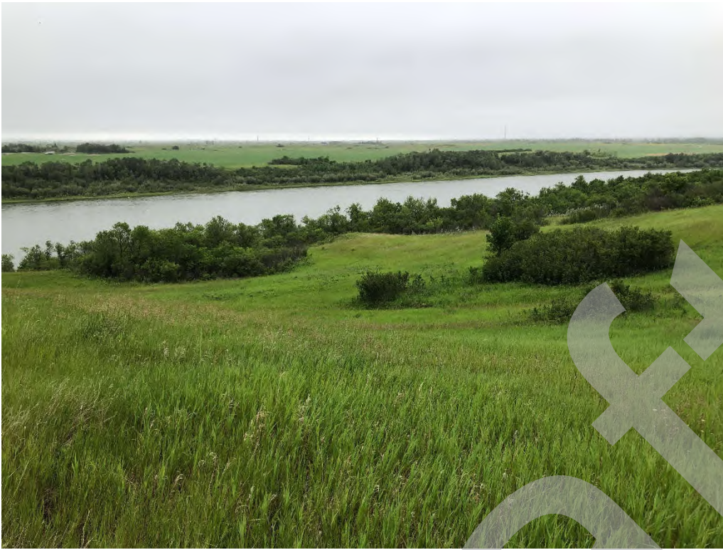
Photo 1 – North side of West Riverbank - Looking down slope at lower slopes of a rotational debris slide (from Field Site 9 of 3D Mapping Figures), looking south.
