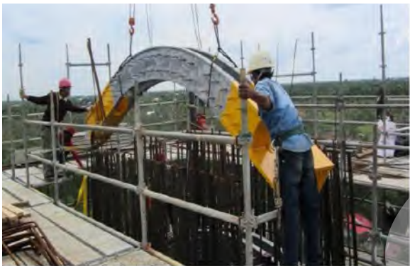
Stay Anchorages Champlain – System Dyna Link form DSI
