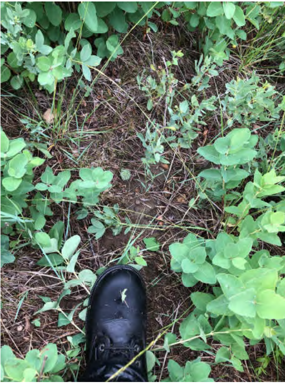
Photo 15 – South side of West Riverbank - Looking at exposed soil between newer vegetation, head scarp of small, recent debris slide (at Field Site 13 of 3D Mapping Figures).
