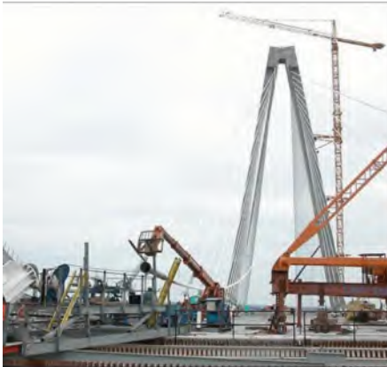
HDPE Duct gets inserted
