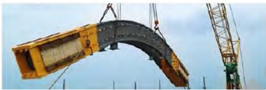
Fig: Dynalink Box Type saddle from DSI – as used at Champlain Bridge
