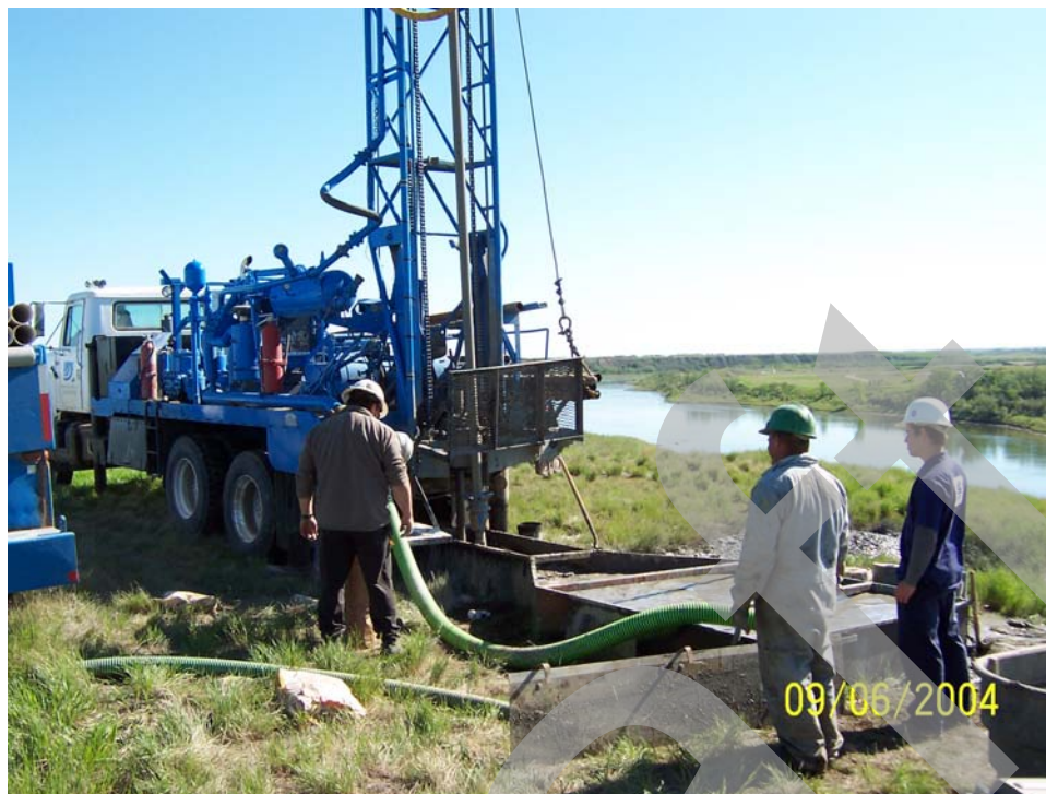
Photograph 3.1 – Failing 1250 hydraulic rotary drill rig utilized for subsurface investigation.
