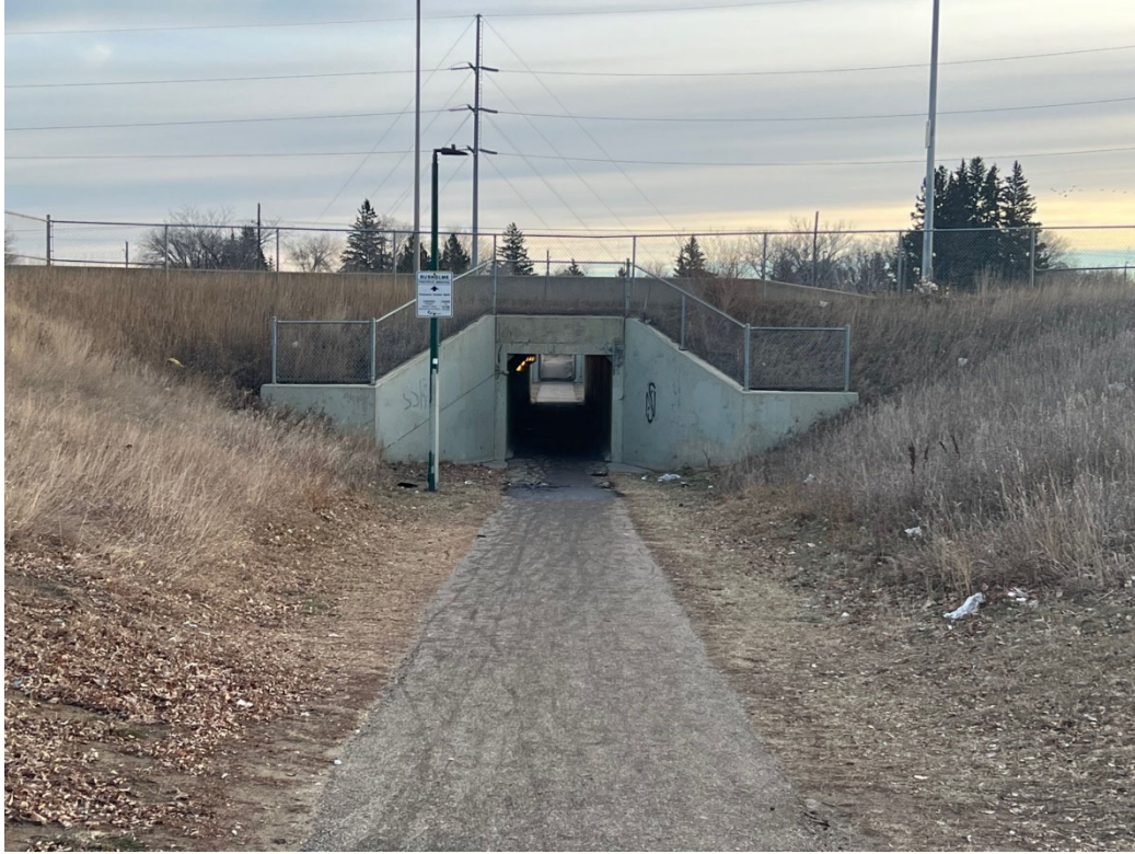
Photograph 7 – Looking easterly (from Confederation Mall side of Circle Drive West)
