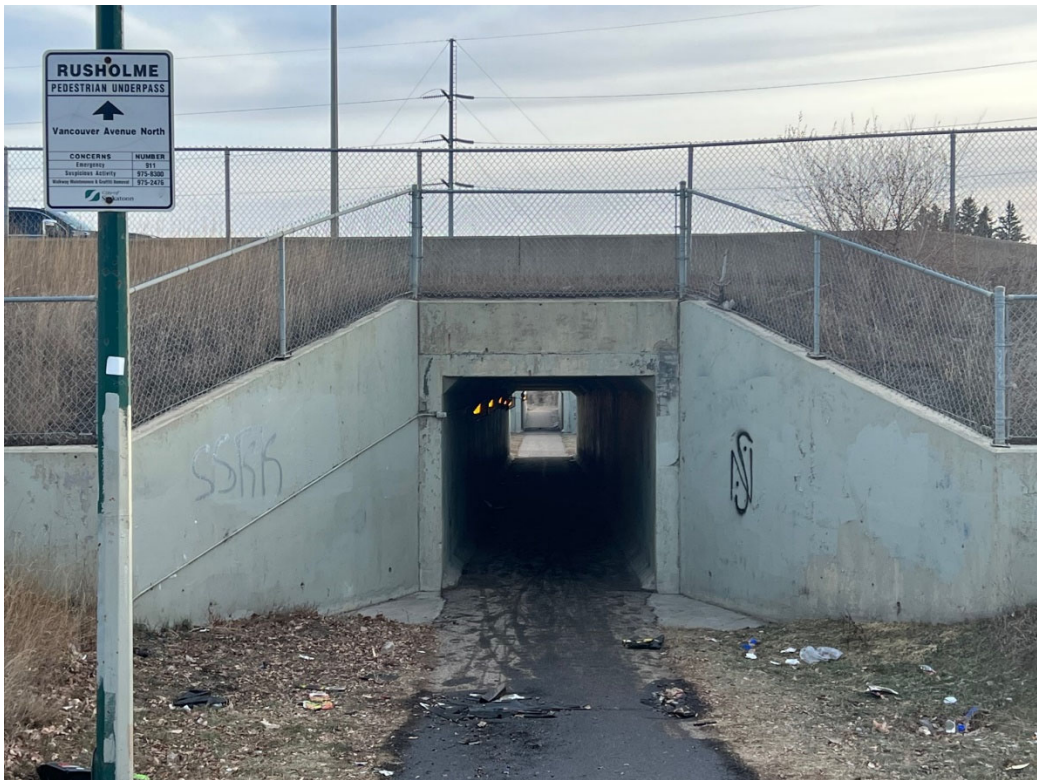
Photograph 8 – Looking easterly (from Confederation Mall side of Circle Drive West)
