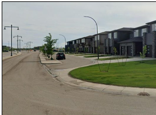
200 block of Brighton Gate, looking east from Dagnone Link intersection Source: Google Maps
