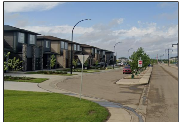
300 block of Brighton Gate, looking west from Dagnone Link intersection Source: Google Maps
