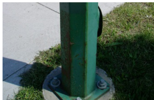
Street Light Pole in Good Condition
