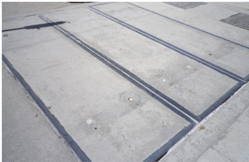
Network Vault Roof in Good Condition
