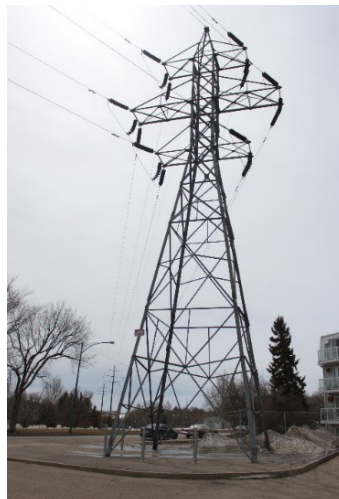
Transmission Tower (Lattice Structure)
