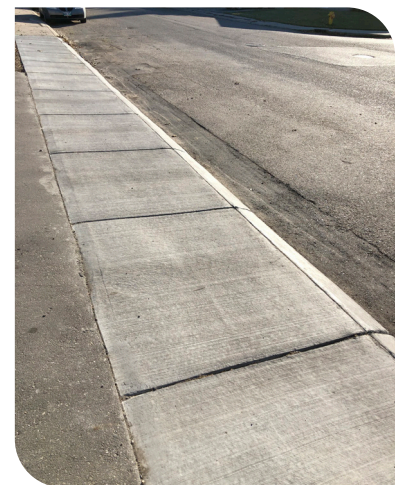
Wollaston Crescent: after
