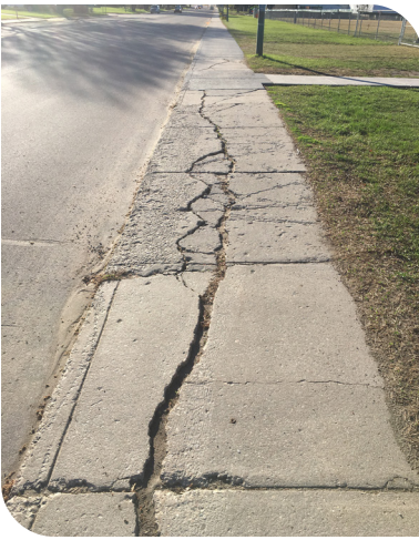
Taylor Street East: before
