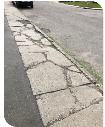
Wollaston Crescent: before
