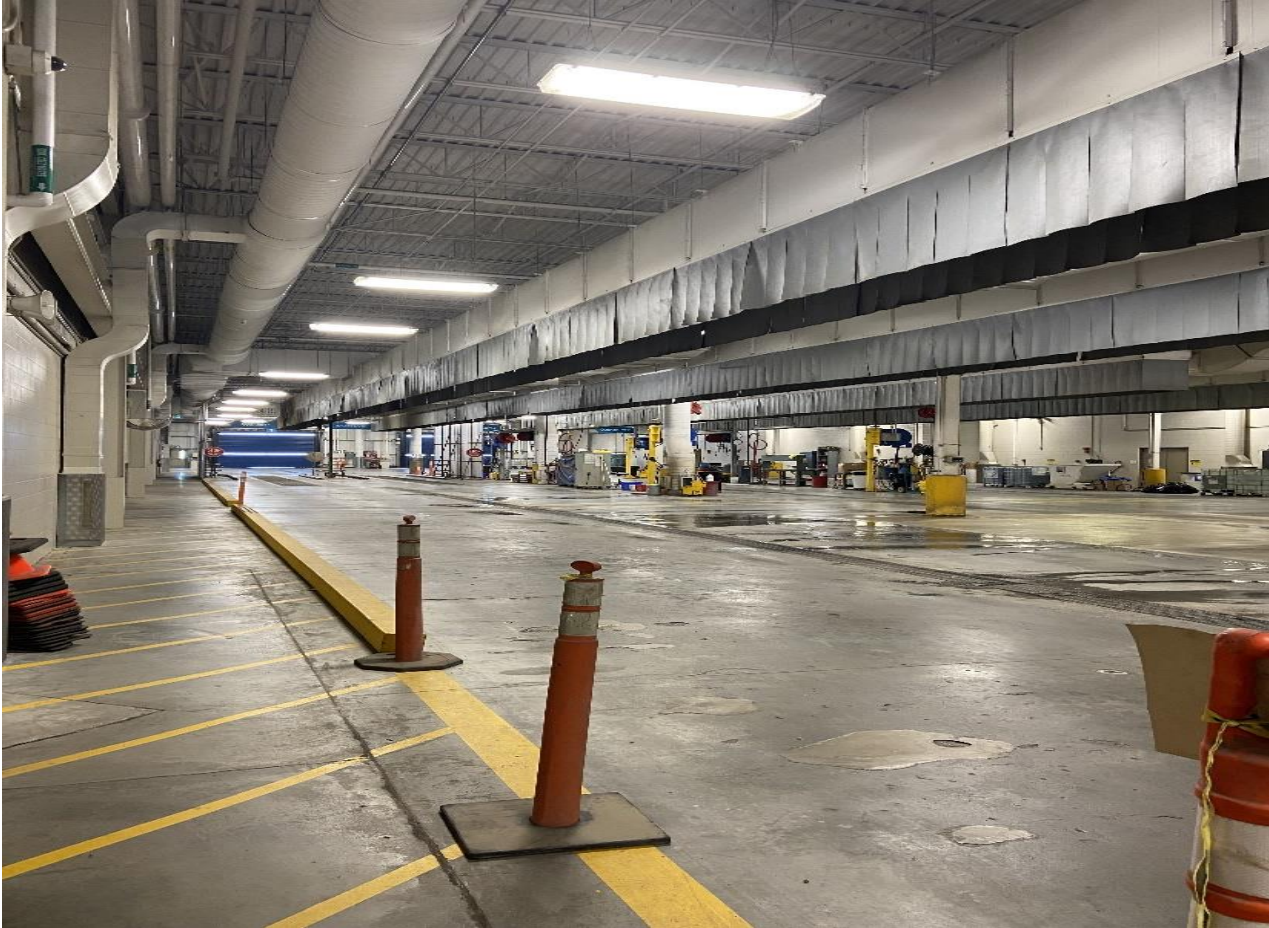
Under-carriage wash area and where the buses first enter the garage
