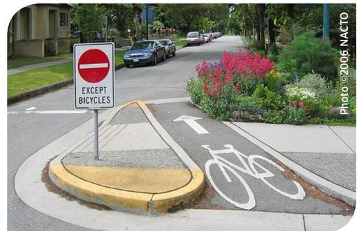
Figure 5.17 - Directional closure in Vancouver, BC
