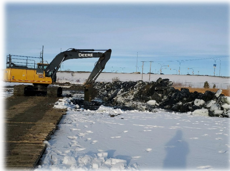
Figure 11: Dredging at Brand Road Storm Pond
