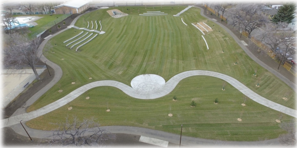
Figure 2: W.W. Ashley Park Substantial Completion Drone Image
