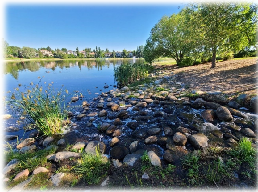
Figure 1: Recirculation Channel at Erindale (John Avant) Pond
