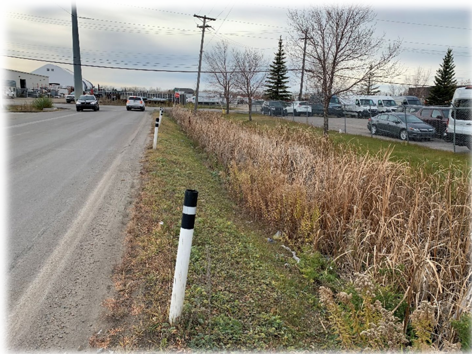
Figure 5: Existing Ditch along Portage Ave
