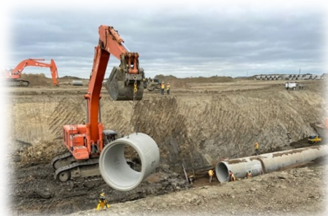
Figure 42: Brighton Storm Trunk Installation
