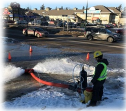
Figure 41: Fire Flow Testing
