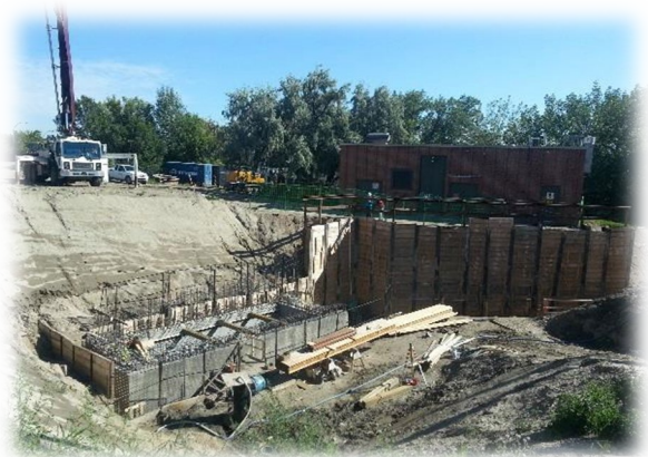
Figure 5: Photograph of Lift Station Infrastructure Construction
