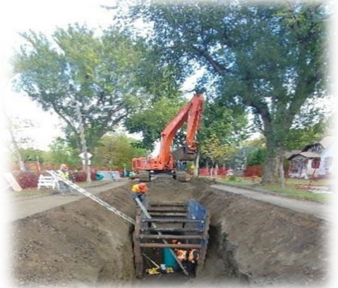
Figure 7: Photograph of Work in an Excavated Trench
