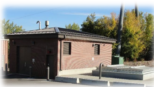
Figure 37: Spadina Lift Station
