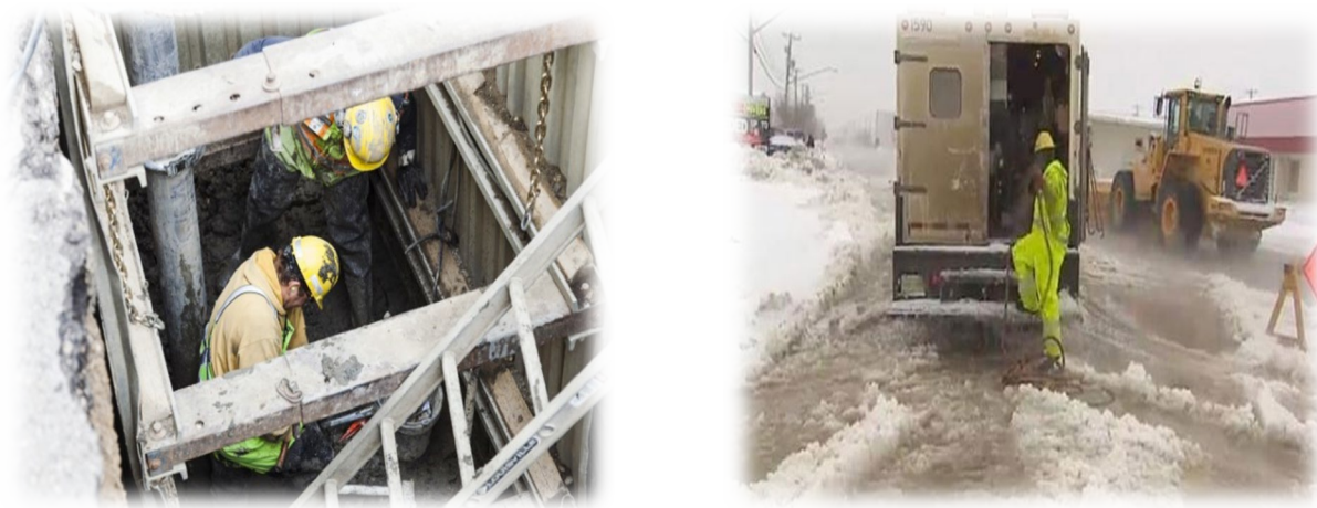
Figure 33: Photographs of Water Main Break Repair Work
