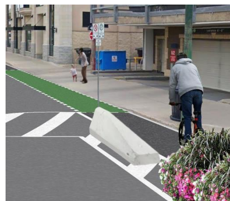
Image 26: Low Profile Transition Barrier at Driveway
