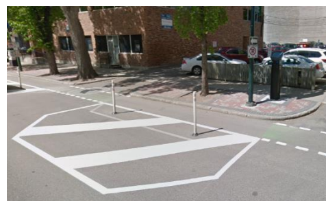
Image 25: Pavement Markings at Driveways Source: Google, Image Capture May 2017
