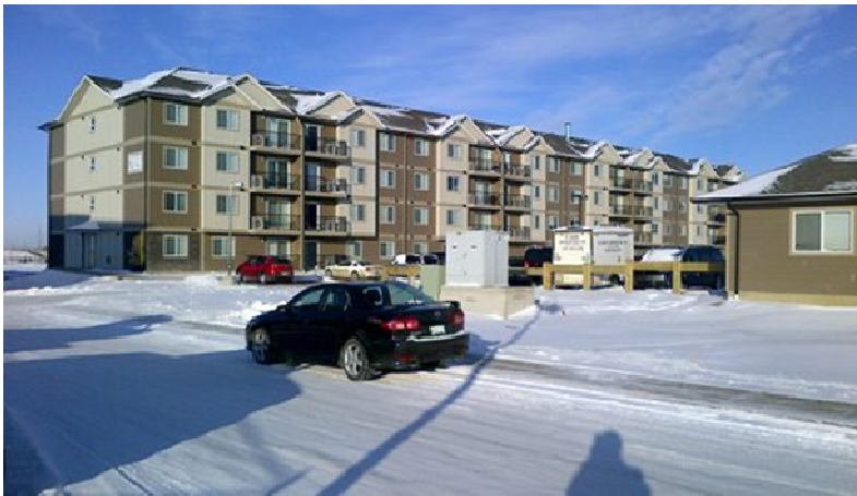
Purpose built rental housing by Broadstreet Properties, Stonebridge neighbourhood
