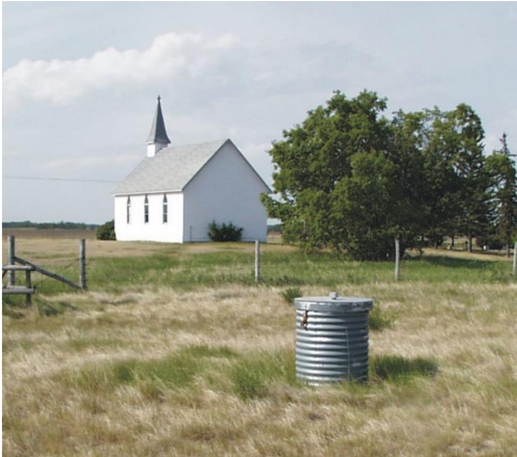
Fig. 1: Large diameter pumping well (source: Water Security Agency)
