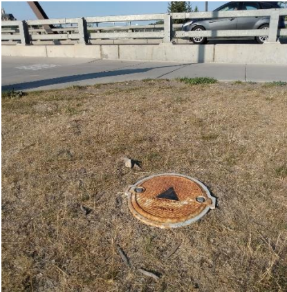
Fig. 2: Flush mounted well
