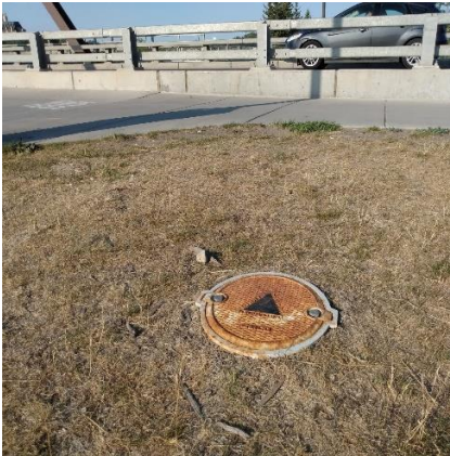
Fig. 2: Flush mounted well
