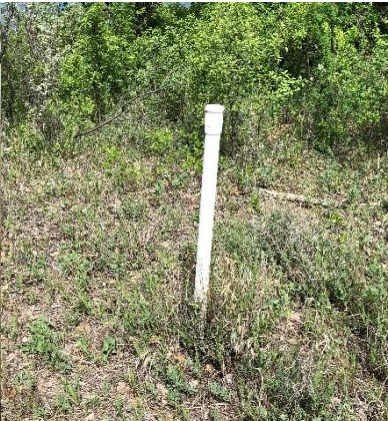
Fig. 3: Well with no protective casing
