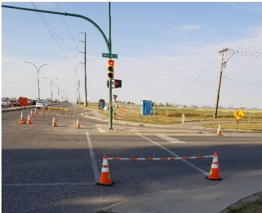
Image 5 and 6: Lack of signage indicating the pathway is closed
