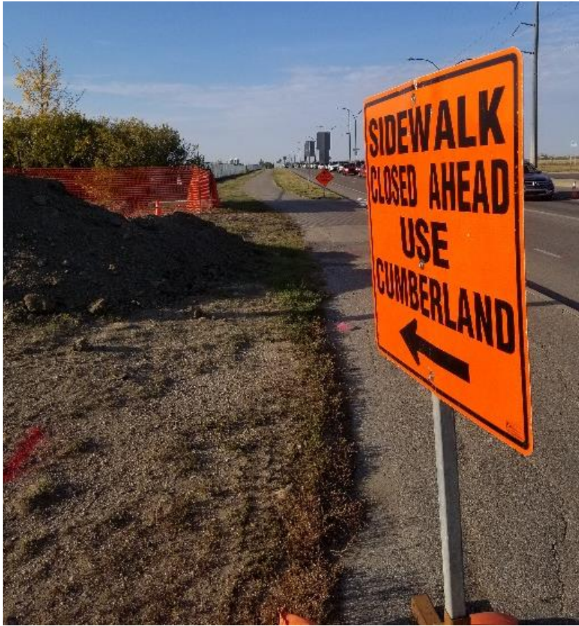
Image 3: Poor orientation of detour sign at Preston Avenue and 14 th Street
