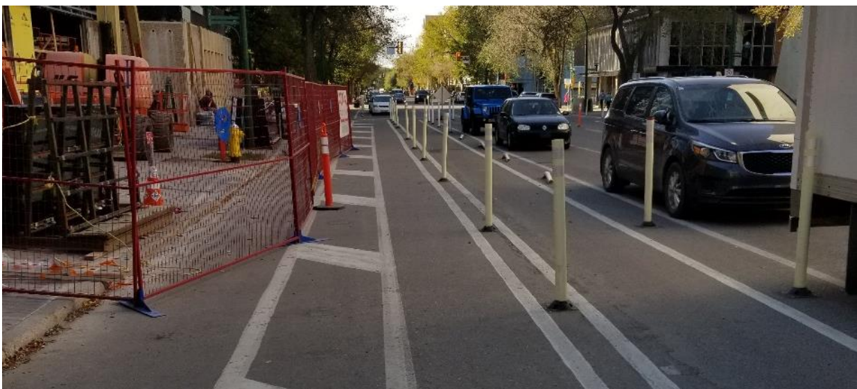
Image 8: Providing a straight, cane detectable edge would improve this diversion for people with visual impairments
