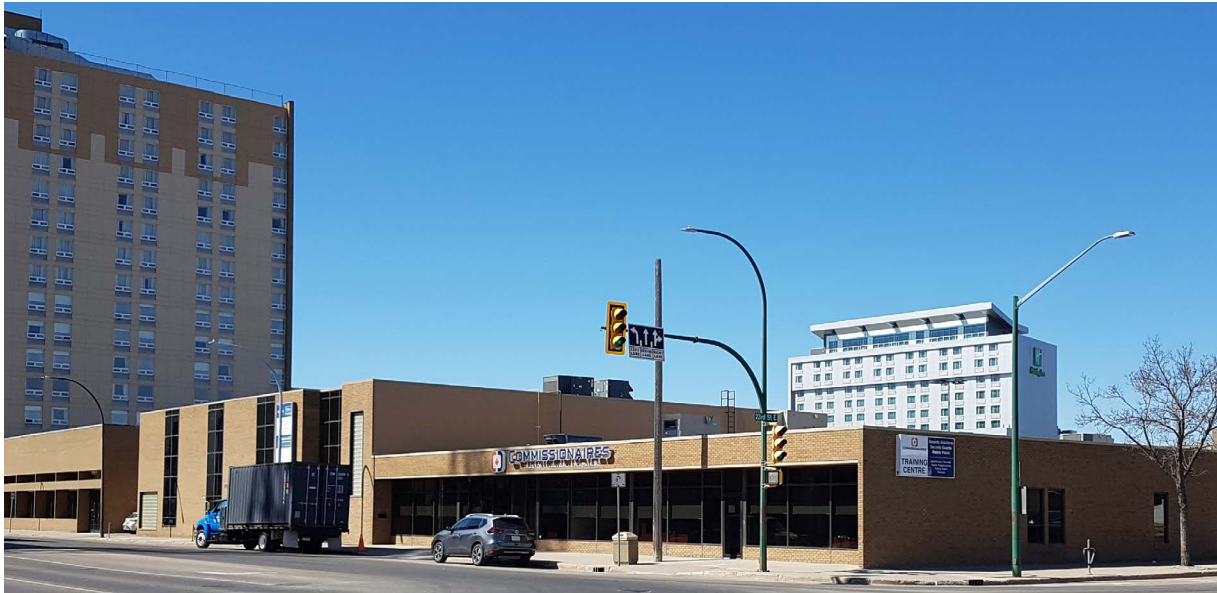
145 - 1st Ave Looking SW from Intersection of 1st Ave & 23rd St
