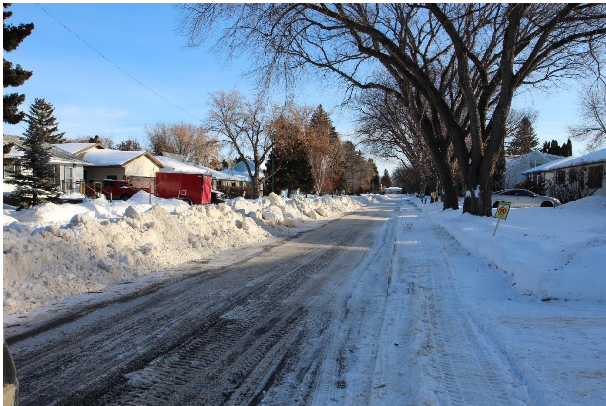
During snow removal process for residential streets: snow is piled in the center of the street before being loaded into trucks
