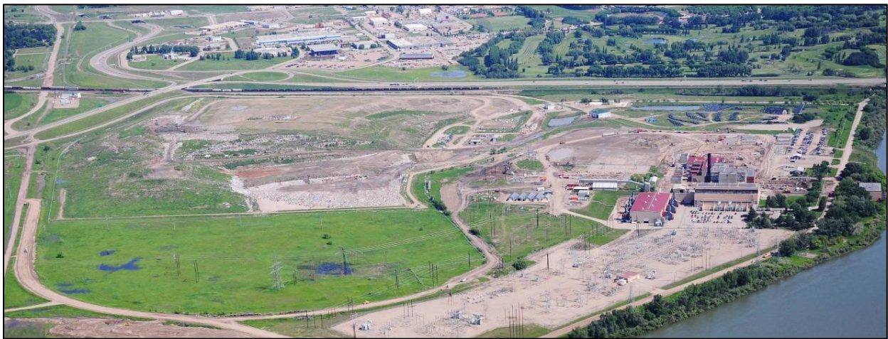
Saskatoon Regional Waste Management Centre
