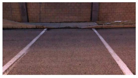
Figure 7-70 Barrier Encroaches on Curb Ramp
