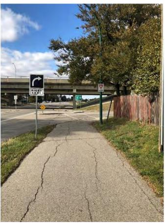
Figure 7-51 Misaligned Curb Ramp
