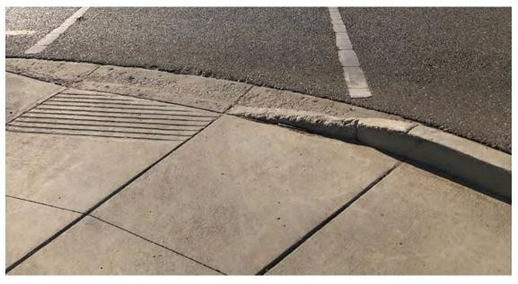
Figure 7-67 Barrier Encroaches on Curb Ramp
