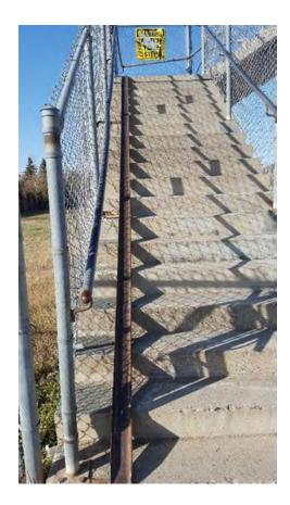
Figure 7-115 Bike Wheel Ramp at Stairs
