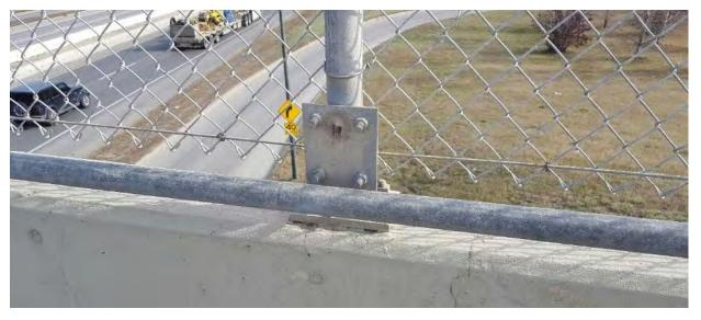
Figure 7-41 Unfastened Handrail
