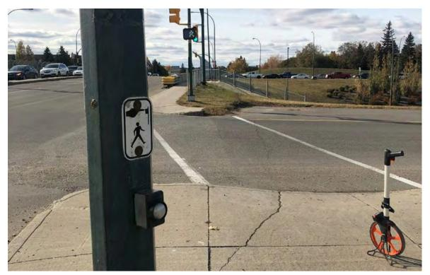
Figure 7-59 Misaligned Pedestrian Recall (looking west, north/south recall)
