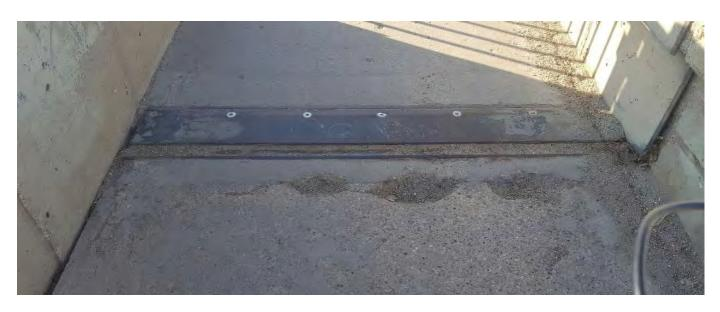
Figure 7-25 Walk Deterioration
