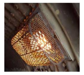
Figure 7-162 Underpass Lighting Reduced Clearance
