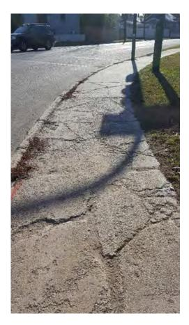
Figure 7-100 Deterioration on Walk
