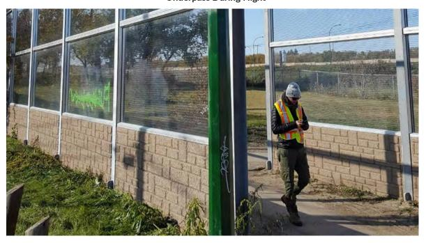
Figure 7-159 Transparent Sound Wall at Switch Back
