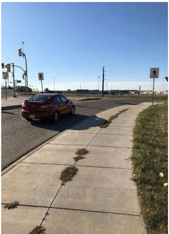
Figure 7-63 Missing Curb Ramps – Dumont Crescent
