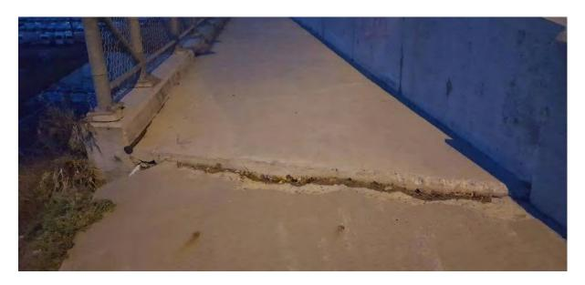
Figure 7-112 Trip Hazard at Deck Transition
