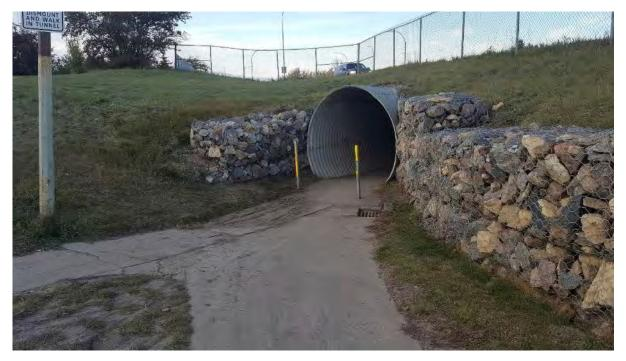
Figure 7-143 Ponding and Bollards at Underpass Entrance
