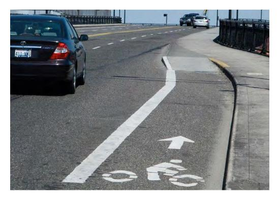
Figure 6-16 Bike Ramp at Bridge
