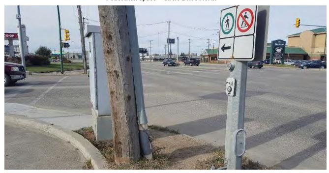
Figure 7-38 Inaccessible Actuated Recall – Avenue C North
