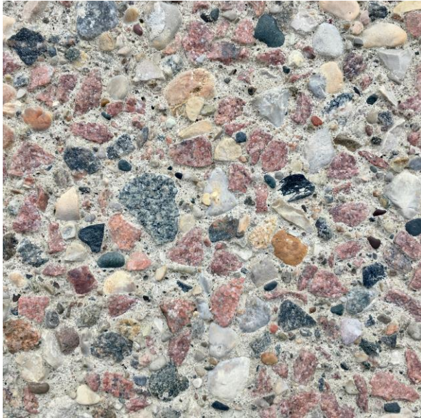
Figure 4: Detail of exposed aggregate concrete.
