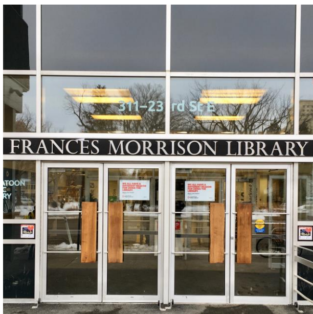
Figure 2: Glazed front entry doors.
