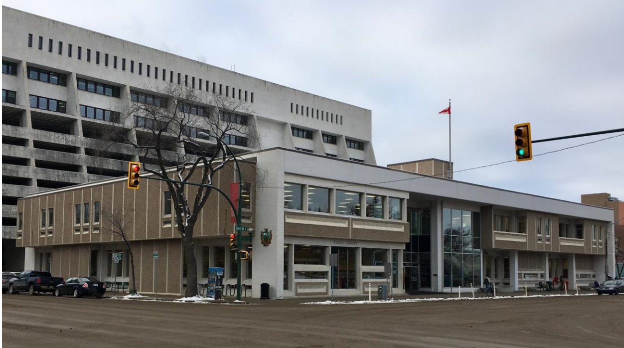
Figure 1: Frances Morrison Library, viewed from the north-east, 2020.
