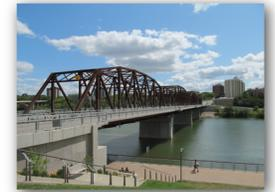
For the next few months, a single span of the historic Traffic Bridge stood alone in the middle of the river. In November, it was lowered to the berm below, cut into smaller pieces and removed, making way for construction of the new bridge.
