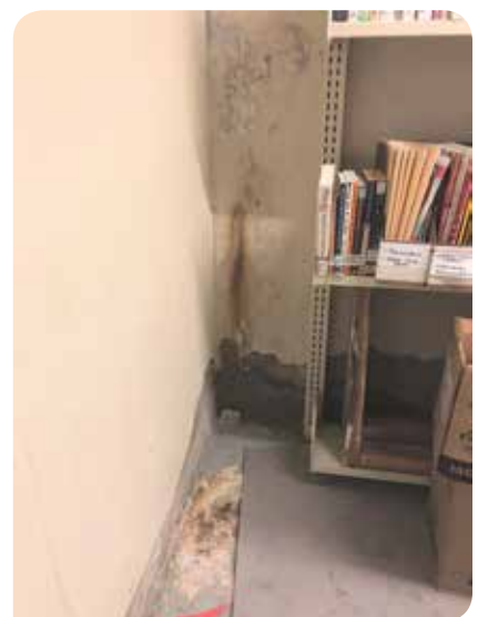
Water damaged and crumbling foundation
