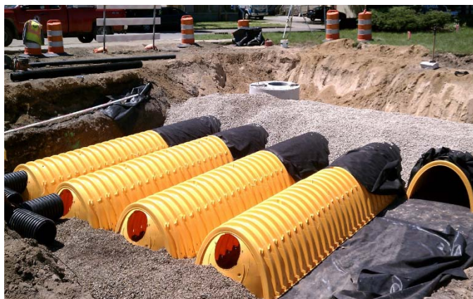
Stormwater Detention System during Installation beneath a Parking Lot. Source: Wikipedia
