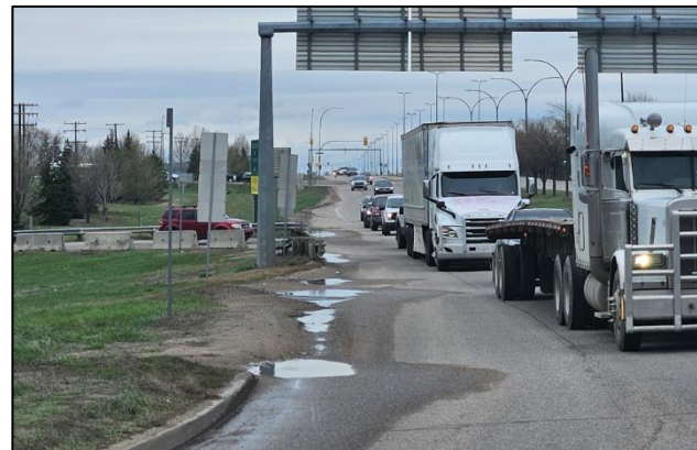
Figure 2-1: Damage to the eastbound shoulder due to vehicles bypassing the vehicle queue
