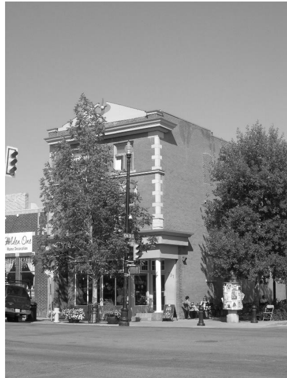
Top: Eaton Block. Source: City of Saskatoon
