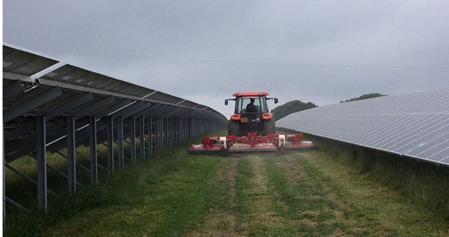
Solar Farm with Naturalized Landscape being mowed
