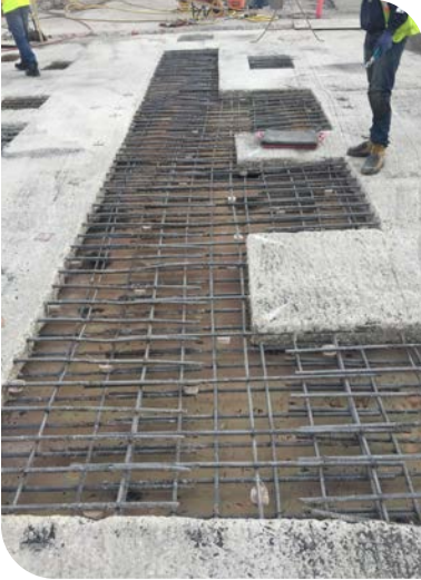
Full depth concrete repairs
