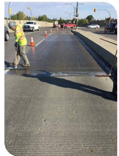
Epoxy crack sealer application on Clarence over Circle Dr Overpass
