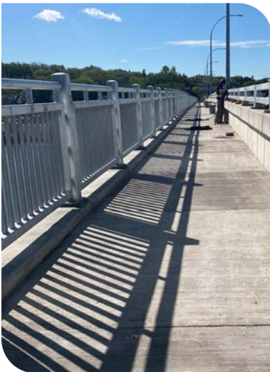
Completed barriers on walkway on Sid Buckwold Bridge rehabilitation project
