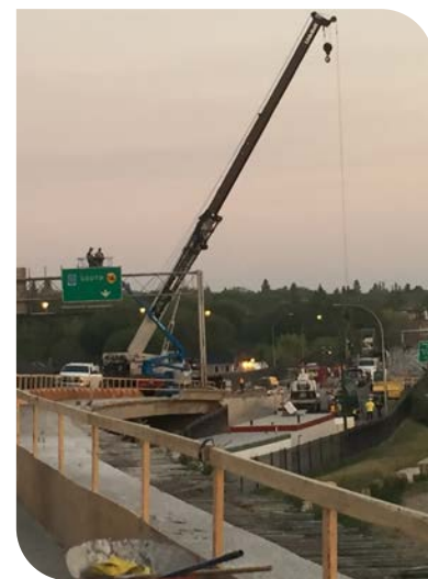
Overhead sign structure removal on Sid Buckwold Bridge Rehabilitation
