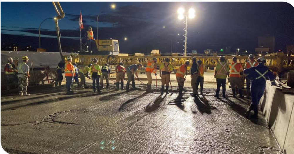
Installation of concrete on Sid Buckwold Bridge
