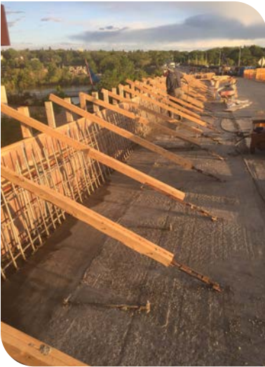
Barrier construction on Sid Buckwold Bridge
