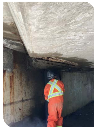
Concrete spall with corrosion on the reinforcing steel
