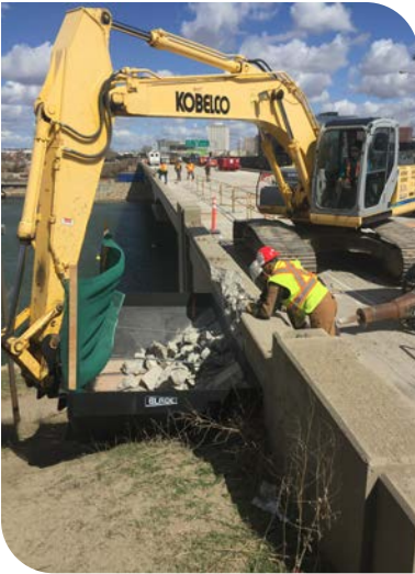
Concrete Barrier Demolition
