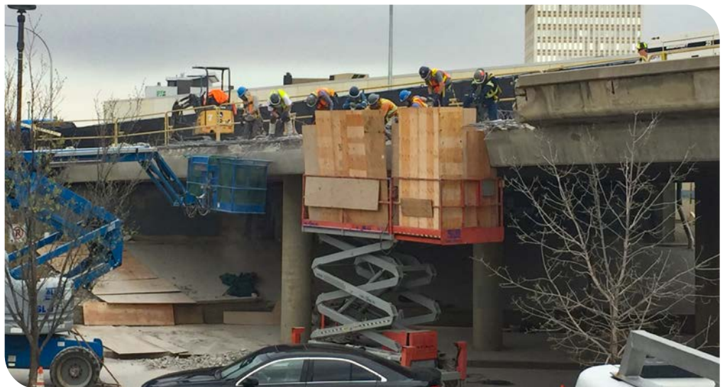
Barrier Demolition on Idylwyld Drive over 19th Street Overpass
