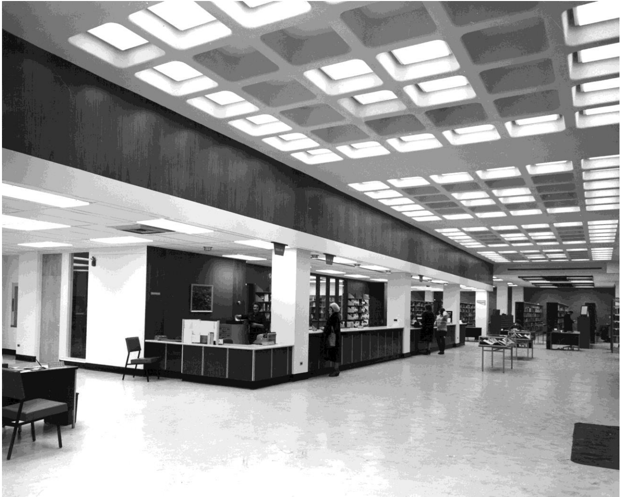
Figure 12: Circulation desk, showing teak wall panelling and waffle slab ceiling, 1966. Photo credit: Lumby Productions Ltd. (SPL Local History Room, PH-88 358).
