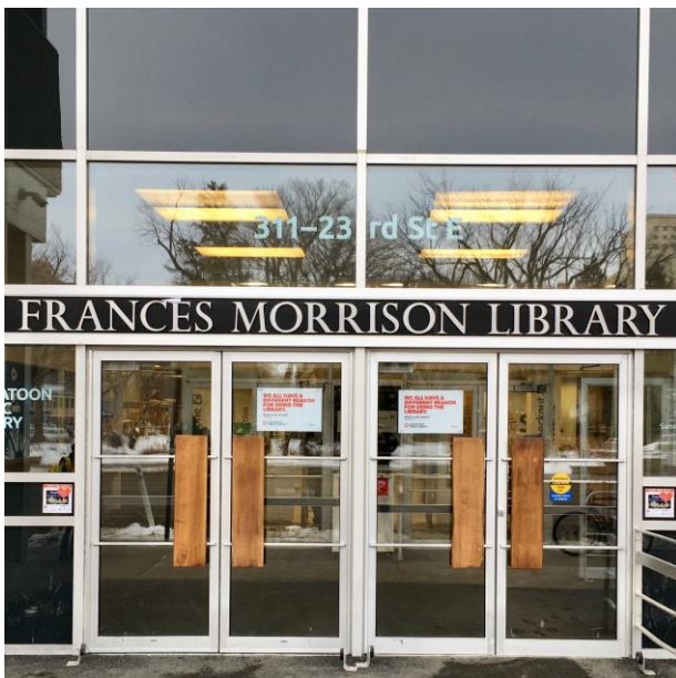
Figure 2: Glazed front entry doors.
